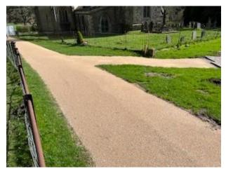
From a brief conversation, construction is apparently with a thick aggregate base using a membrane of Non-woven geotextile fabric and Malvern(?) as a top layer. The finish is designed with a camber so surface water falls either side. Timber edging is sometimes used.
